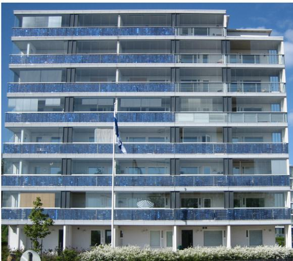
**Figure 1** Solar panels, integrated in a block of flats in the Latokartano ecological housing area (Helsinki, Finland). [https://upload.wikimedia.org/wikipedia/commons/6/66/Solar\\_panels\\_integrated\\_in\\_a\\_block\\_of\\_flats\\_in\\_Vuikki\\_Helsinki\\_Finland.jpg](https://upload.wikimedia.org/wikipedia/commons/6/66/Solar_panels_integrated_in_a_block_of_flats_in_Vuikki_Helsinki_Finland.jpg) Credit: Pöllö.
